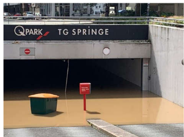
Figure 11: Flooded car park in Hagen, Germany
