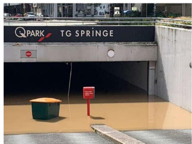
Figure 11: Flooded car park in Hagen, Germany
